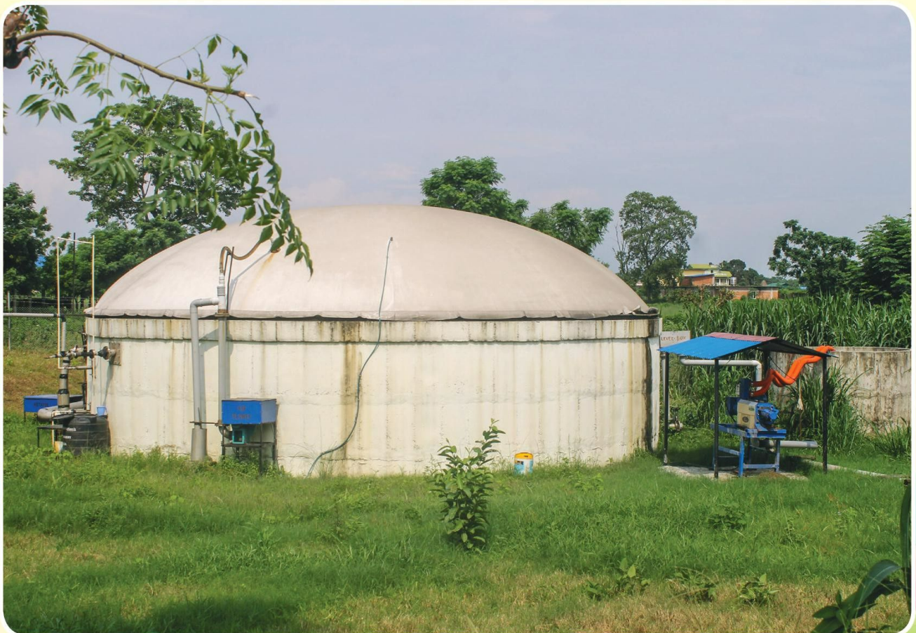
Biogas Plant with Solid Liquid separator
